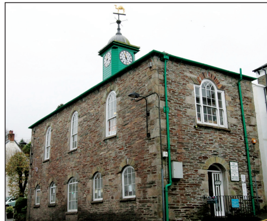
Fig 19. Windvane in the shape of a one humped camel on the old Town Hall, Camelford. Source: Photograph by the Author.
